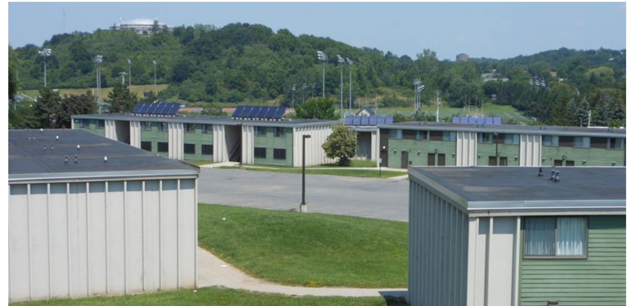
SOLAR PANELS INSTALLED ON THE ROOFS OF SOUTH CAMPUS TOWNHOUSES SUPPLY 50 PERCENT TO 60 PERCENT OF THE ENERGY NECESSARY TO HEAT THE WATER FOR THE RESIDENTIAL UNITS. ©2000-2015 ZACKIN PUBLICATIONS INC.
