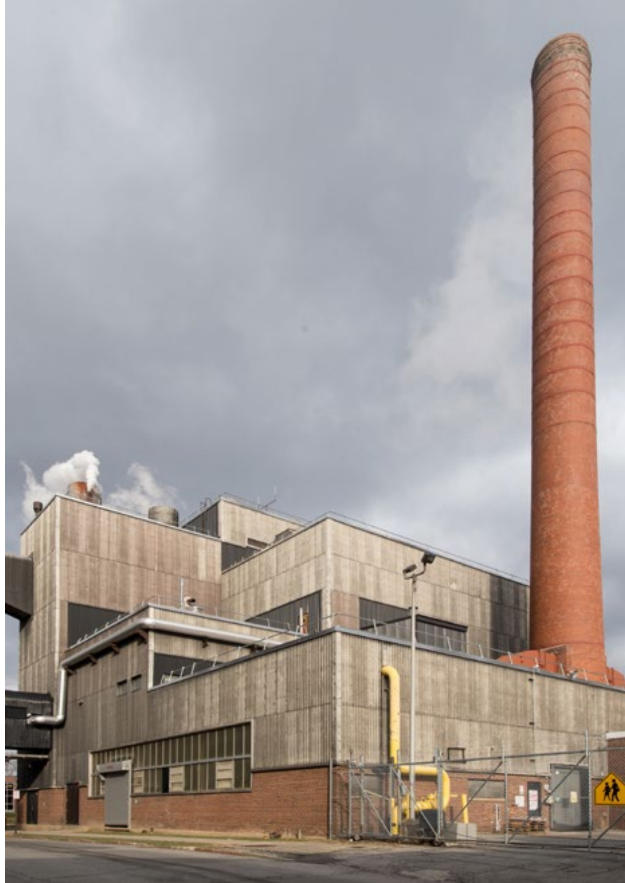
EXISTING ENERGY PLANT
