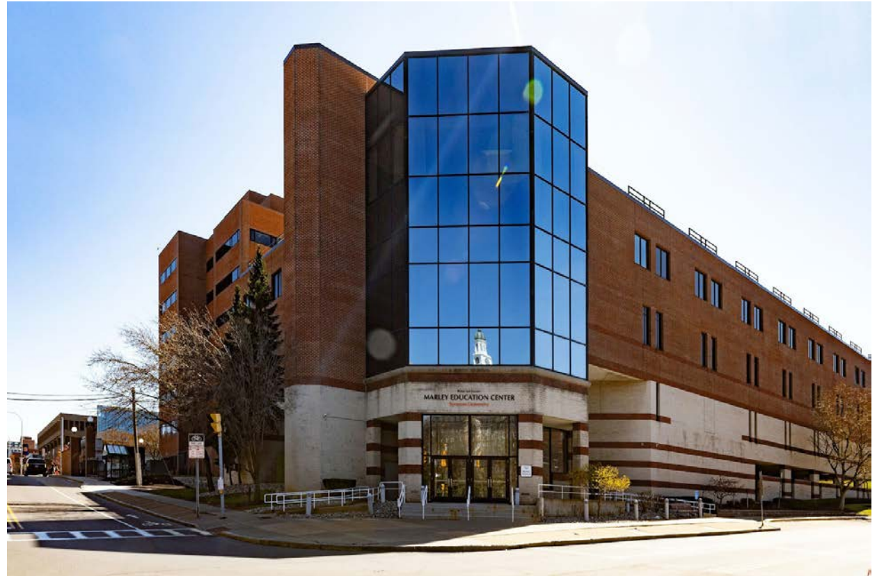
MARLEY BUILDING EXISTING CONDITION
